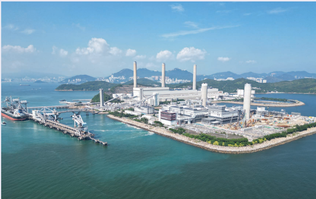
Lamma Power Station, HK Electric
