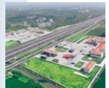
Shanghai-Hangzhou Expressway Jiaying Section
