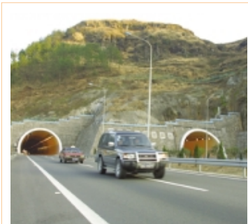
Shangsang Expressway Panlongling Tunnel No.1 & No.2
