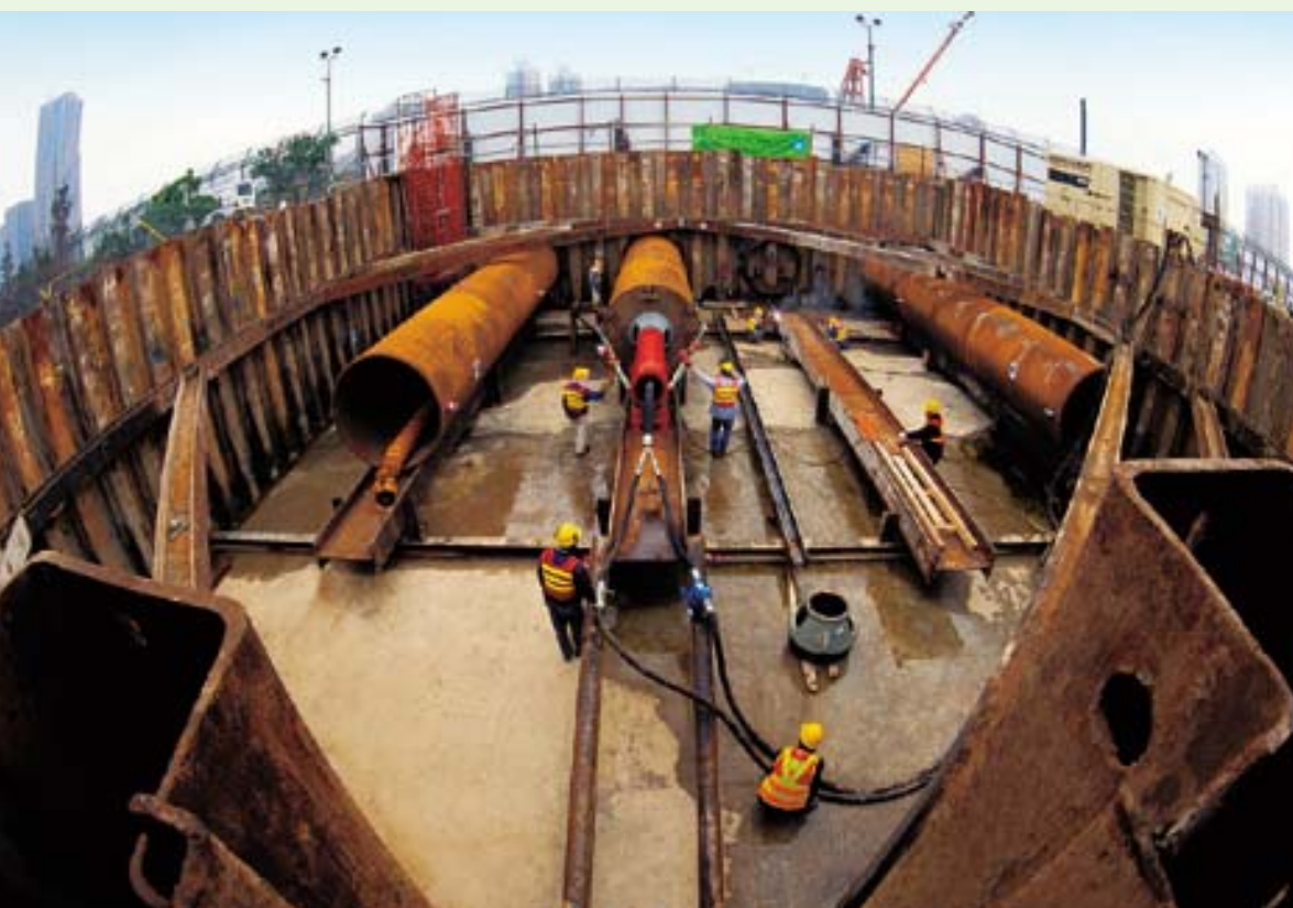
U-Tech's trenchless technology for pipe-laying greatly reduces disturbance to the public and the environment. Here, engineers use pipe ramming to lay 1,800 mm-diameter pipes in Lok Ma Chau, the largest such project in Hong Kong.
