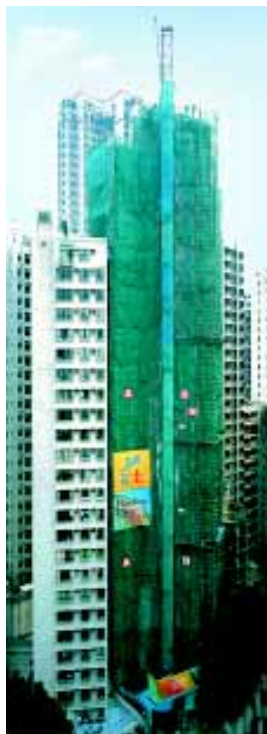
Reading Place, Mid-level (construction works in progress)
