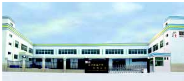
Yuanzhou plant extension
