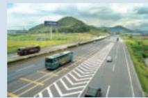
A 122.8km closed system asphalt-paved dual three lane expressway running between Huanggang in Shenzhen and Guangdan in Guangzhou where it connects to the ESW Ring Road.
