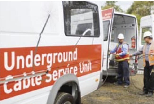
CitiPower and Powercor took the lead in introducing technology that accurately pinpoints the location of an underground cable and minimises the area needed to excavate to repair a fault.
