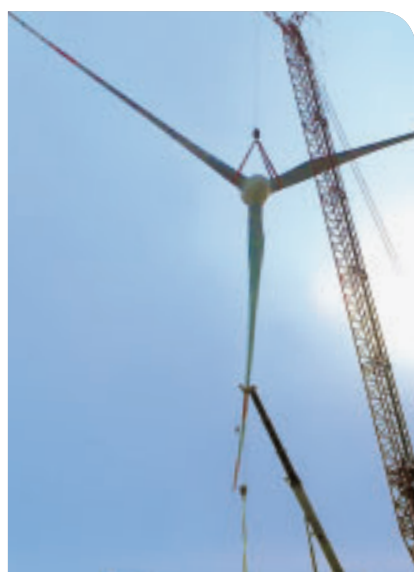
○ Blade-raising at Qian'an, CLP's first wholly-owned wind farm in China
