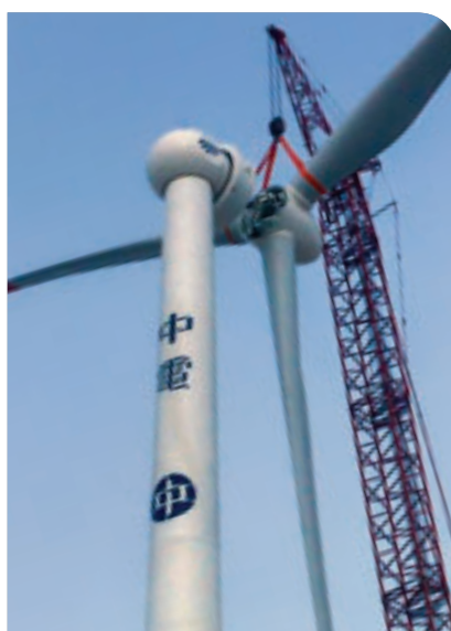
○ Blade-raising at Qian'an, CLP's first wholly-owned wind farm in China
