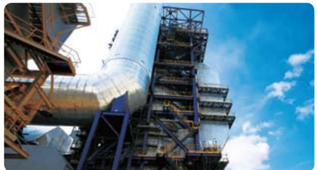
An FGD plant and a Low NO<sub>x</sub> Burner system have been installed for the coal-fired generating unit L5.
