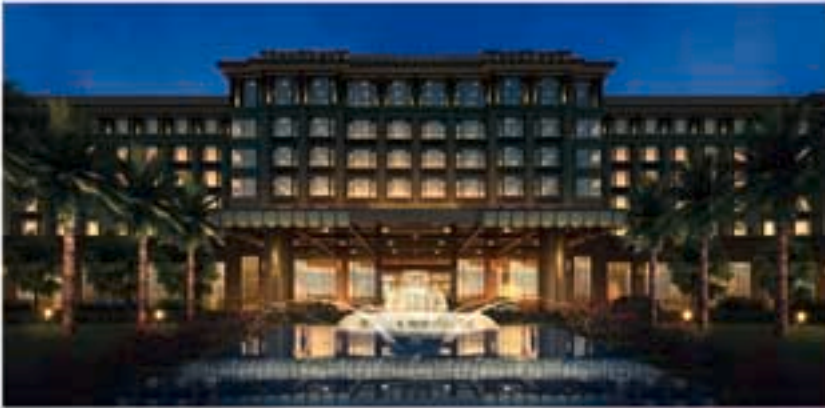
REGAL YUHONG HOTEL (2012) ZHENGZHOU ■ MAINLAND CHINA
