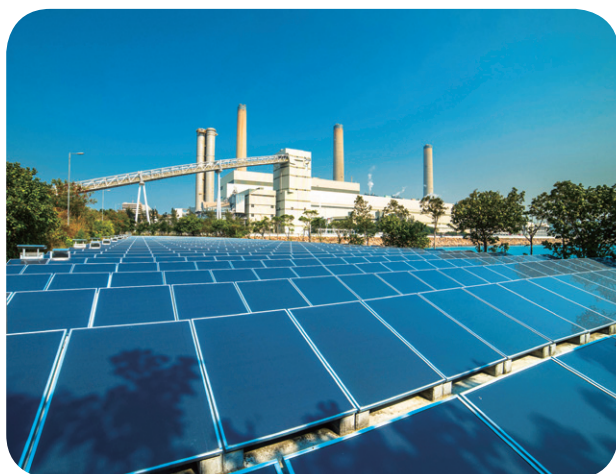
The solar power system makes use of rooftops and open space at Lamma Power Station.
