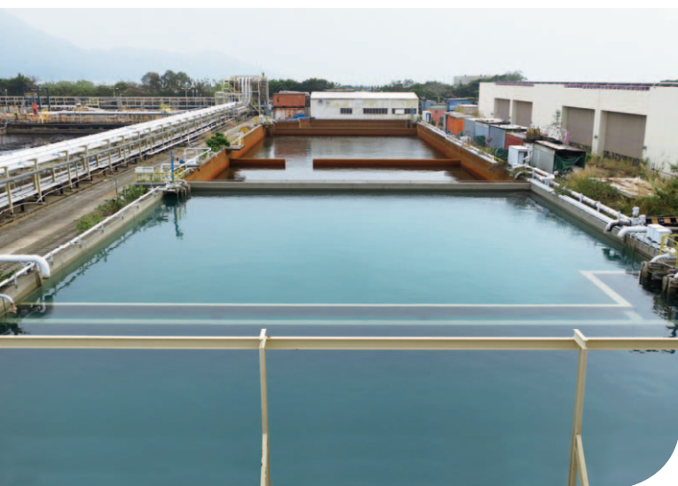
Reservoir for recovered waste water and rain water at Lamma Power Station.
