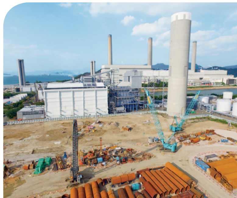
Construction in full swing for the new L10 gas-fired generating unit.
