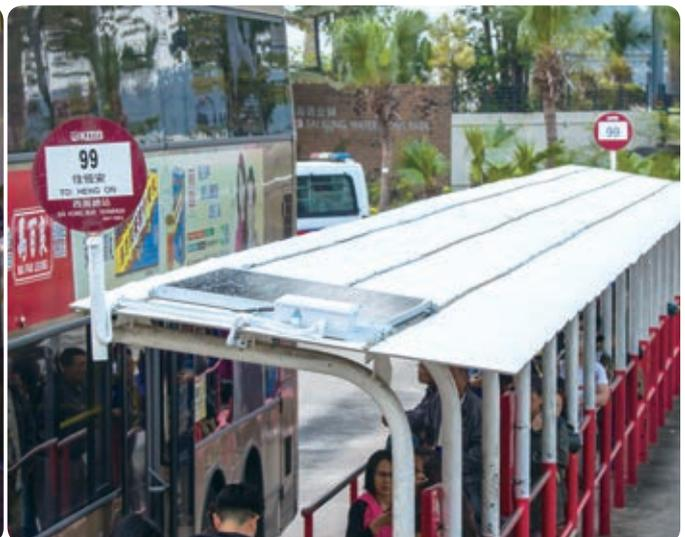
100 bus stops have been equipped with solar power equipment
