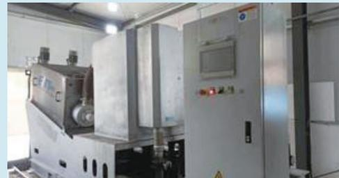
Picture: New sewage desludging system
