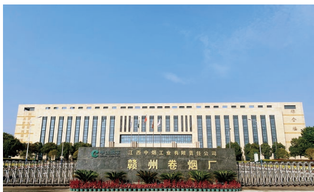
贛州中煙捲煙廠項目 Ganzhou Zhongyan Cigarette Factory Project
