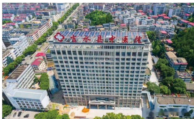
吉安吉水縣中醫醫院項目 Ji'an Jishui County Chinese Medicine Hospital Project
