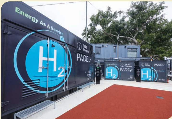
The Group's Modular Hydrogen Power Generation System is a pilot project now underway at a recreational venue in Sai Kung, where it will provide electricity and hot water.
