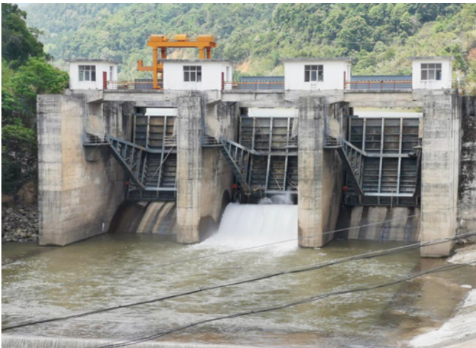
Yunnan hydropower plant revitalized with support from Guangdong Branch
