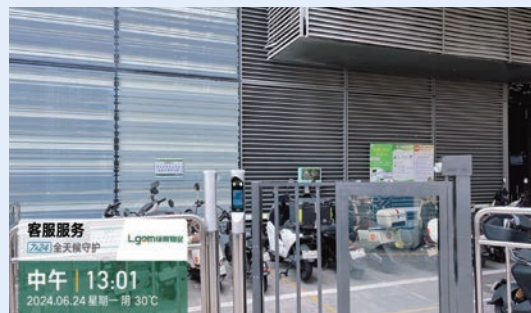
Installation of Facial Recognition System in Residential E-bike Parking Areas 住宅電動單車停放區增設人臉識別
