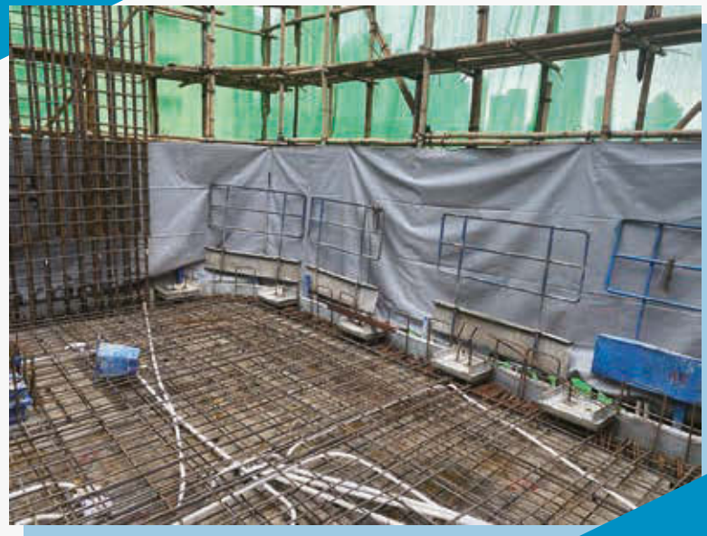
■ Noise barriers hang on the hoarding 於圍板繫上隔音屏障
