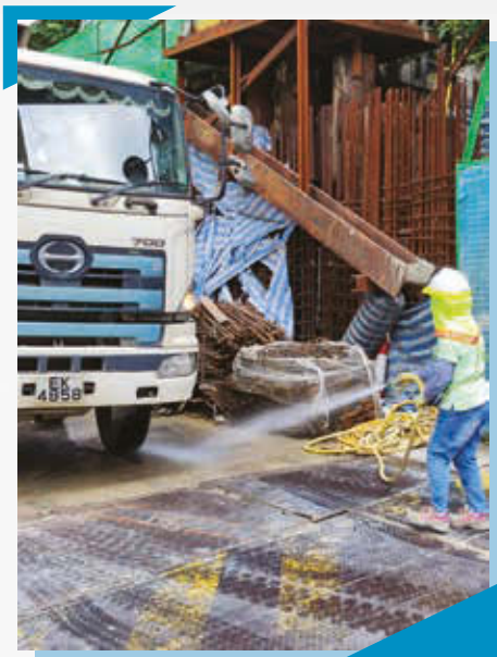
Designated wheel washing area at site 於地盤設立指定輪胎清洗區
