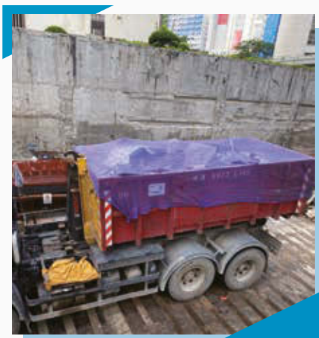
Materials covered with tarpaulin sheets 用防水布覆蓋物料
