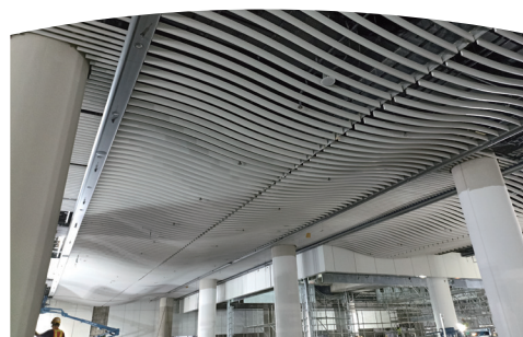
HKIA Terminal 2 Expansion Works – Design, supply and installation of lower-level baffle and external ceiling system 香港國際機場二號客運大樓擴建工程－設計、供應及安裝低層天幕及室外天花系統
