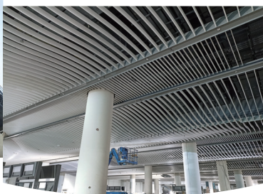
HKIA Terminal 2 Expansion Works – Design, supply and installation of lower-level baffle and external ceiling system 香港國際機場二號客運大樓擴建工程－設計、供應及安裝低層天幕及室外天花系統
