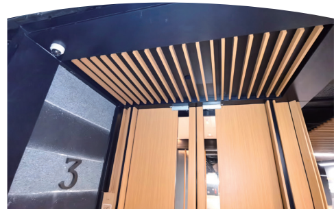
Ho Man Tin Station Package One Property Development – Supply and installation of baffle ceiling at LG1 and LG2 carpark 何文田站第一期物業發展項目－供應及安裝地下1層及地下2層停車場天花
