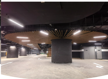
Ho Man Tin Station Package One Property Development – Supply and installation of baffle ceiling at LG1 and LG2 carpark 何文田站第一期物業發展項目－供應及安裝地下1層及地下2層停車場天花
