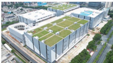
7 Shenzhen Pingshan Project
