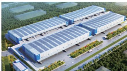
14 Foshan Gaoming Project#
