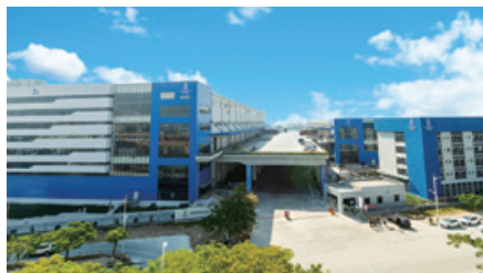
12 Foshan Nanhai Project
