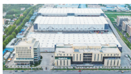
42 Zhengzhou Erqi Project
