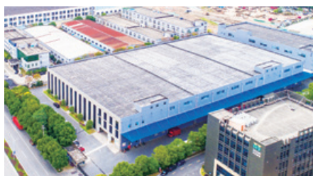
5 Shanghai Qingpu Project
