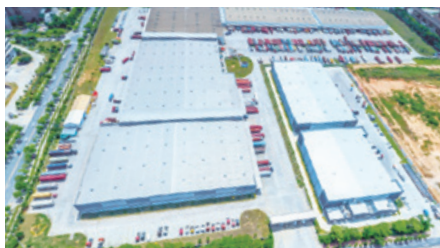
8 Shenzhen Pingshan East Project
