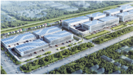
19 SZI Beijing Southwest Integrated Logistics Hub (Phase I) Intelligent Logistics Center #
