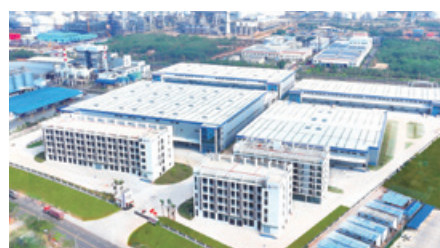
39 Hainan Yangpu Project
