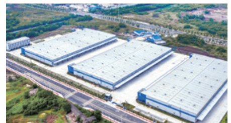
33 Chongqing Shuangfu Project
