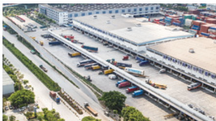
4 SZI Western Logistics Park
