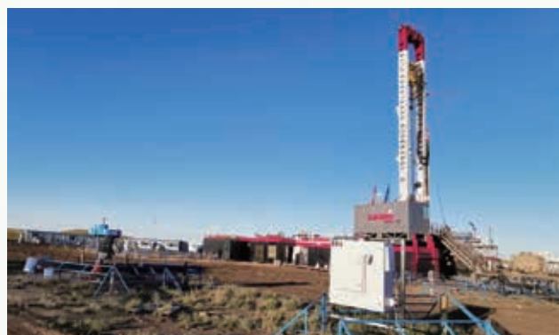
Drilling rig for new wells drilling
