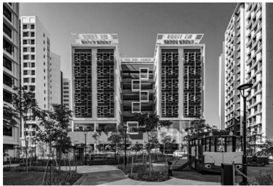
Nursing Home at the East Region
