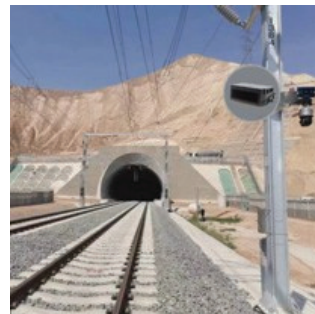
Installed over train tracks
