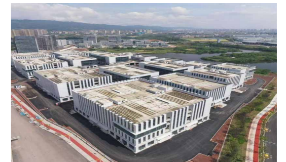
Partial View of the PPP project—the Tuanjiehu Big Data Intelligent Industrial Park in Jiangjin District
