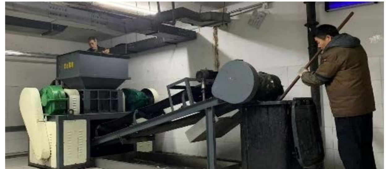
Garbage Crushing Equipment Upgrade at Qingpu Wuyue Plaza
