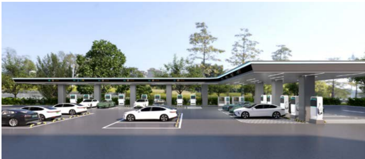
Photovoltaic-Storage-Charging Integrated Charging Station at Nanjing Jianye Wuyue Plaza
