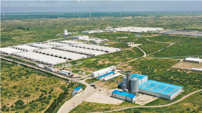
After the construction of Naiman Muyuan Farm 5
