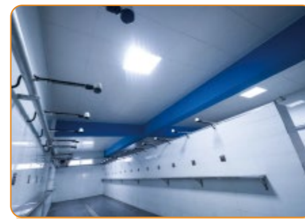
Renovated and refreshed bathrooms
