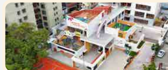
Aerial View of the Kindergarten in Lishi Town, Shaoguan City
