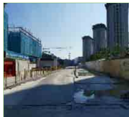
Construction vehicle washing passage
