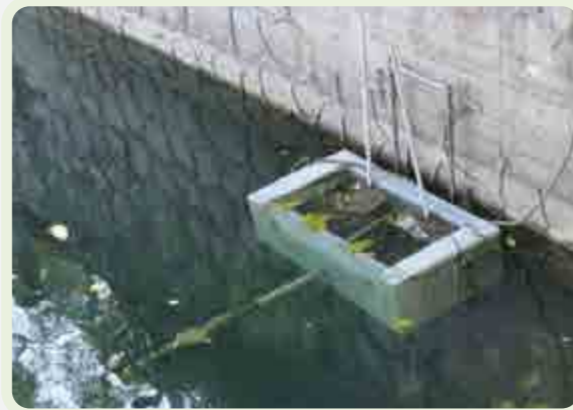
Self-developed water surface garbage collection stations automatically collect floating debris and other water surface garbage
