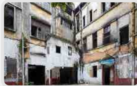
Zhongshuge Bookstore Before Renovation
