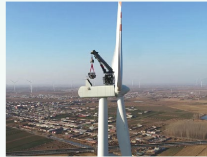
The UTC600 self-climbing crane in operation
