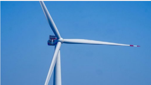
“Qihang” 20 MW Floating Offshore Wind Turbine
