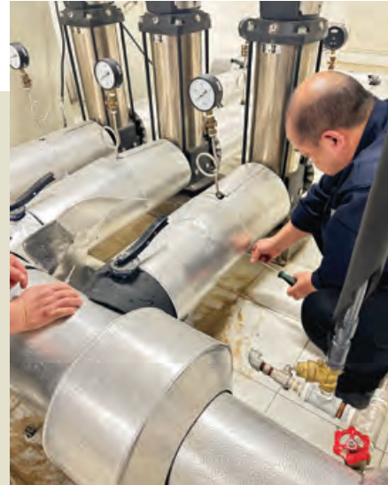
Engineers inspecting the water pumps and air conditioning system at GHB
