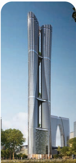
Suzhou China State Construction International Fortune Center Ultra-Low Energy Project
