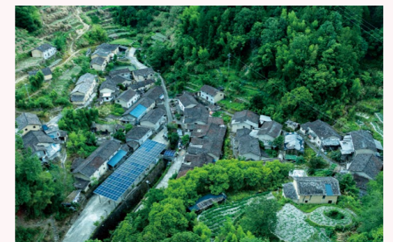
Rooftop Photovoltaic Assistance Project in Huangyu Village, Qingyuan County, Zhejiang
