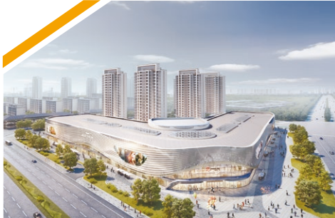
WUXI YIXING POWERLONG PLAZA
