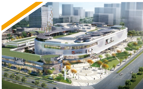
JINGDEZHEN POWERLONG PLAZA
