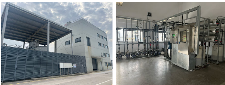
Wastewater Treatment Plant
