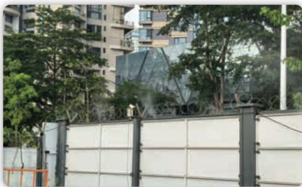
Sprinkling system surrounding construction zone
