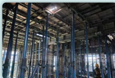
Aluminium formwork
