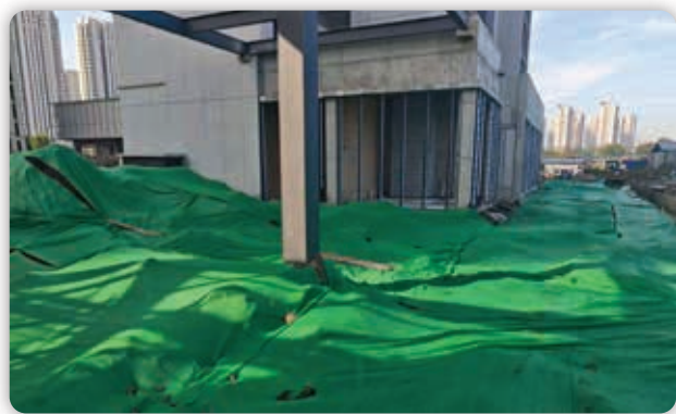
Covering of exposed earth
