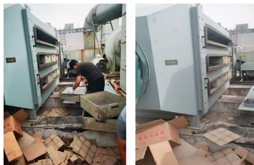
Exhaust Outlet Testing and Exhaust Gas Treatment Equipment Upgrades and Maintenance
