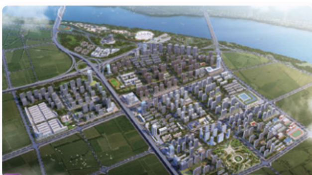
39 Housing and Infrastructure Construction Project, Qian Shi Hou Shi Sub-area, Lanshan District, Linyi, Shandong Province
