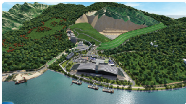
1 West New Territories Landfill Extension
