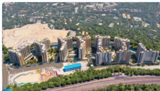
8 Construction of Public Housing Development at Kam Sheung Road Site 1 Phase 1 and 2, Yuen Long
