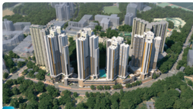
12 Public Housing Redevelopment at Mei Tung Estate (Older Part)
