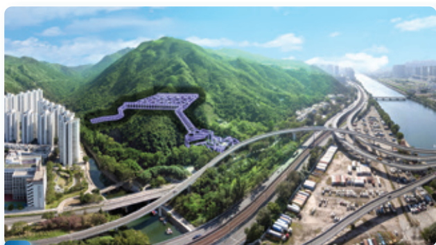
3 Relocation of Sha Tin Sewage Treatment Works to Caverns – Main Caverns Construction
