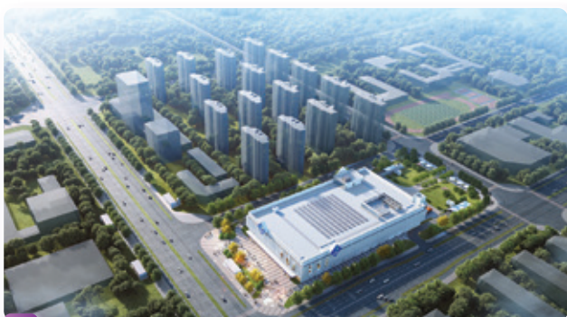
30 Housing Construction Project, Hefei Economic Development Zone, Anhui Province
