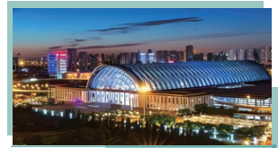
Tianjinxi Railway Station
