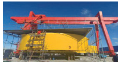
◆ An Underwater Data Server Room Construction Project
