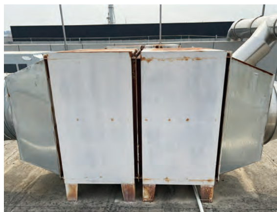
Low temperature plasma waste gas treatment equipment 低溫等離子廢氣處理設備
