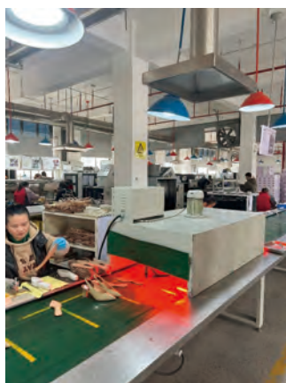
Workshop VOC collection equipment 車間VOC收集裝備
