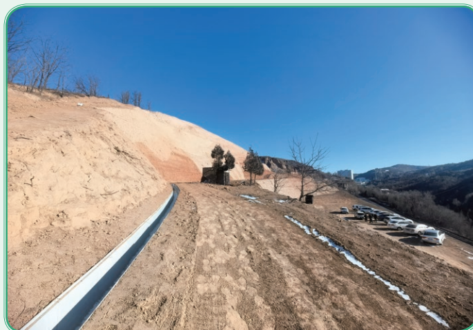
Picture: Geological Disaster Management Project in Hejiashe Village Coal Mining Subsidence Area 圖：賀家社村採煤沉陷區地質災害治理工程項目
