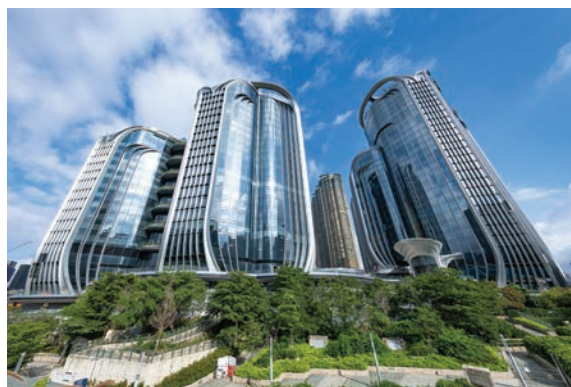
Curtain Wall Project of International Gateway Centre
