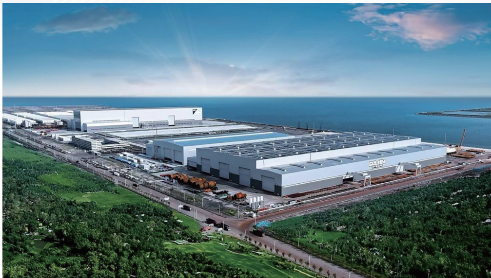
Dajin Heavy Industry Hebei Tangshan Caofeidian Deep-sea Offshore Facility
