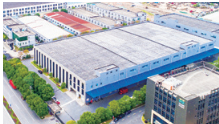
5 Shanghai Qingpu Project
