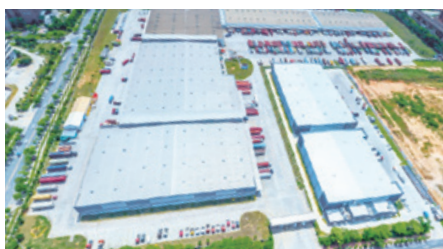
8 Shenzhen Pingshan East Project
