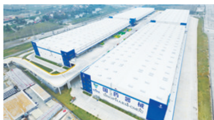
17 Foshan Gaoming Project
