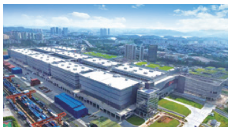
1 Shenzhen International Integrated Logistics Hub Center
