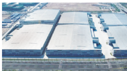
34 Chongqing Shapingba Project
