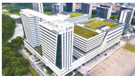
6 Shenzhen Liguang Project
