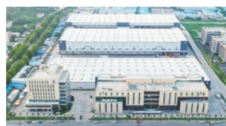
42 Zhengzhou Erqi Project
