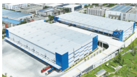
37 Chengdu Wenjiang Project
