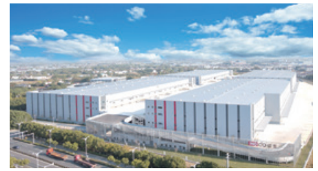
9 Wuxi Xishan Project
