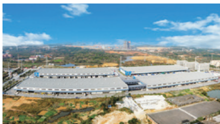
26 Nanchang Jingkai Project
