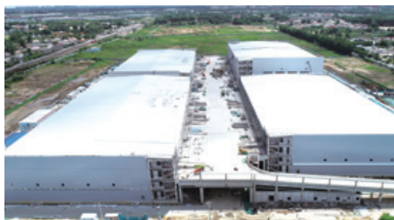
19 SZI Beijing Southwest Integrated Logistics Hub Intelligent Logistics Center
