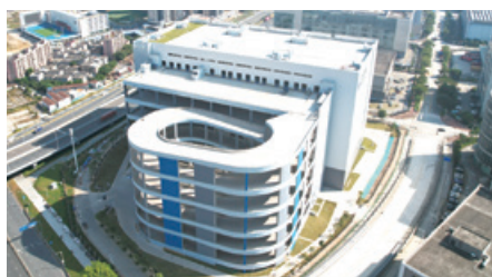
9 Shenzhen Yantian Project
