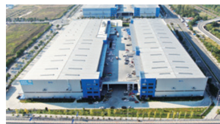
36 Chengdu Qingbaijiang Project
