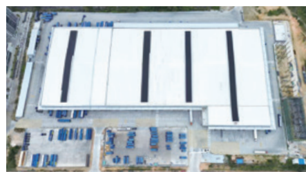
18 Huizhou Dayawan Project
