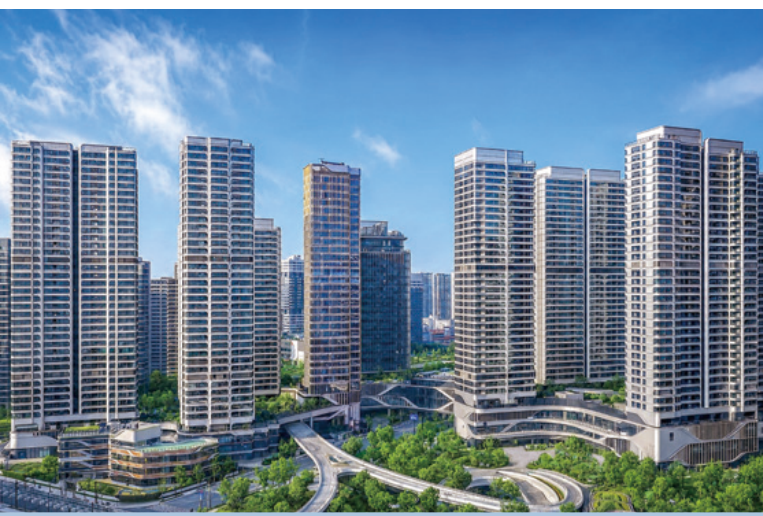
○ Hangzhou IFC Mansion, Hangzhou
